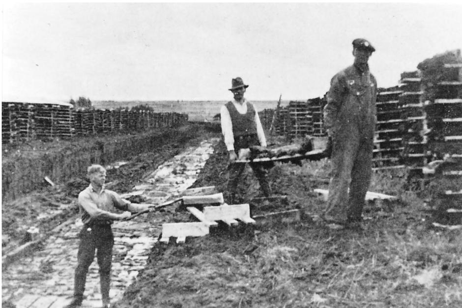
Figure 2. Block-cut mining activities in the Isle-Verte peatland, 18 km east of Ca-couna bog, Québec, during the 1940s. The mining trench is bordered by two baulks where peat blocks were deposited for drying (from Risi and others 1953; courtesy of Ministère des Ressources naturelles du Québec).
