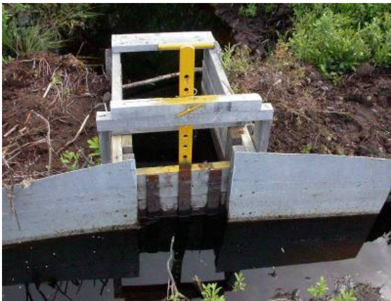
6a. Water level control (barrier).
