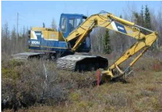
4a. Cleaning drainage ditches.
