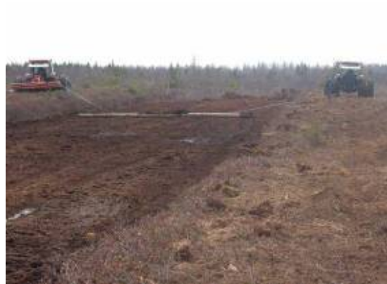
4f. Basin leveling using a wooden pole pulled by two tractors.
