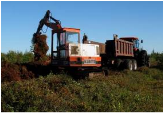
4c. Removal of surface vegetation.
