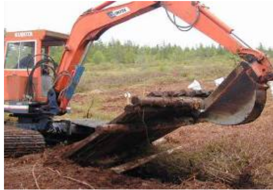
4b. Culvert installation.
