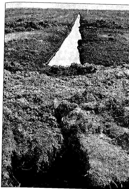
Fig. 2 Peat dam used to block drainage ditches
