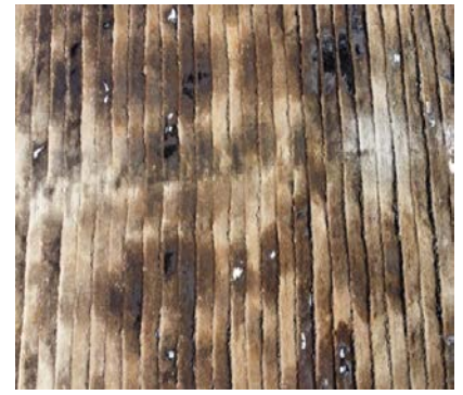
C. In Progress
