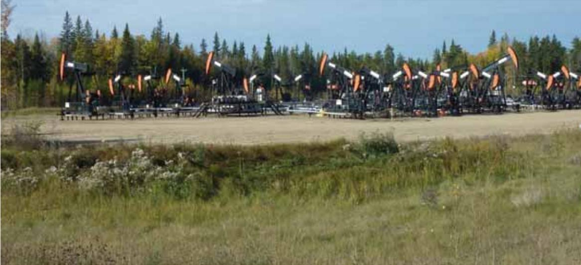
*Figure 0.1 In situ oil sands well pad made of compacted mineral fill situated within a mosaic of boreal forest and wetland ecosystem. This well pad in the Cold Lake Oil Sands region is sized approximately 1.8 ha and supports 27 well heads, each one connected to an oil pump (“pumping jack”).*
