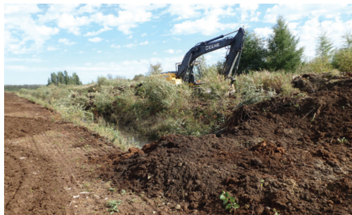
Figure 6. Removing the embankment and filling the ditch at Elma in Manitoba.
