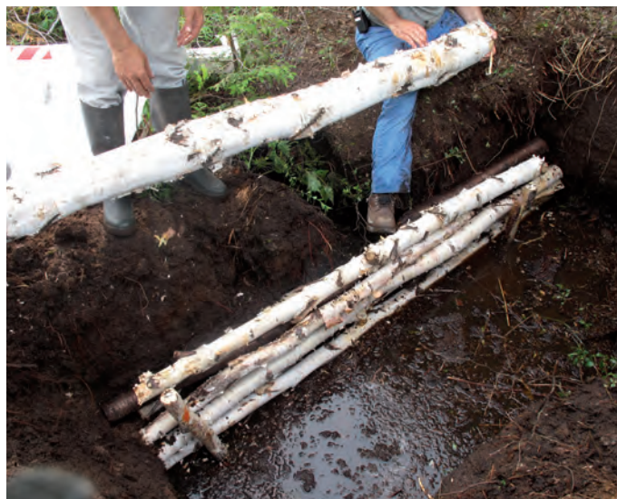
Figure 25. Dam made of wooden logs: a technique which is not recommended.
