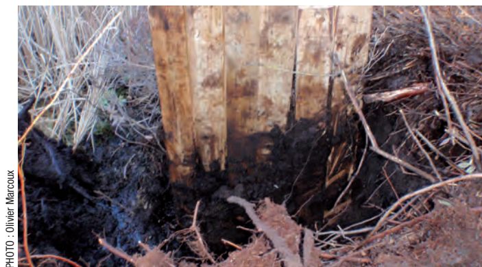
Figure 26. The technique of a vertical dam by individual insertion; observation of the openings between planks.
