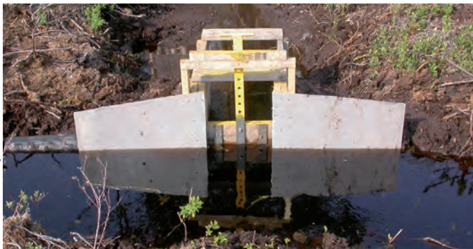
Figure 33. Regulation tank being controlled from above (1 st photo), installed to block a basin in Sainte-Marguerite peatland, in Québec. A regulation tank controlled from below (2 nd photo), installed to block a basin in Shippagan (New Brunswick).
