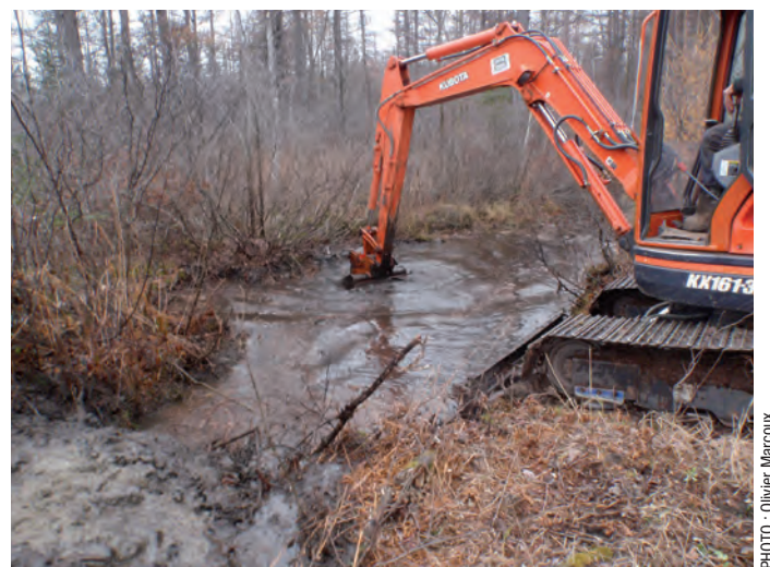
Figure 34. Creating a pool allows for the collection of peat material for the construction of a peat dam at the Grande plée Bleue peatland (Québec).
