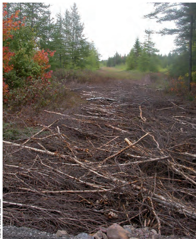
Figure 17. Road covered with wood logs and branches to allow for passage of the machinery in the peatland Grande plée Bleue (Québec).
