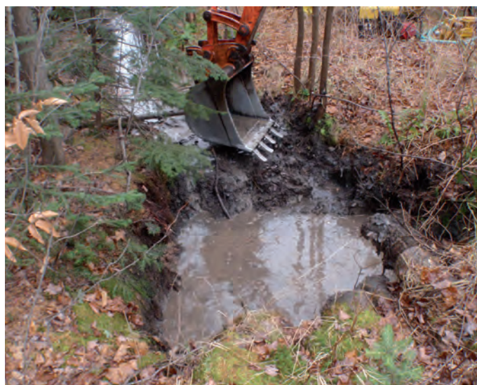
Figure 23. Peat dam in construction at the Grande plée Bleue peatland (Québec).
