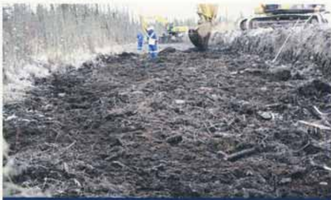
FIGURE 1. COMPLETE REMOVAL OF CLAY PAT WITH FLUFFING/DECOMPACTION.
