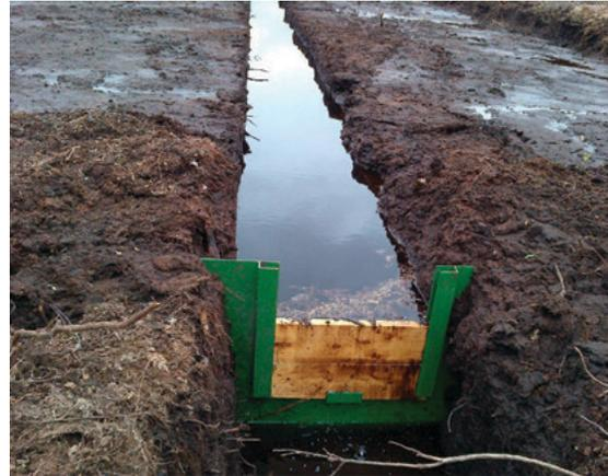
**Figure 16.** Fixed dam where the maximum water level is adjusted by adding or removing boards in a steel plate with a bracket.
