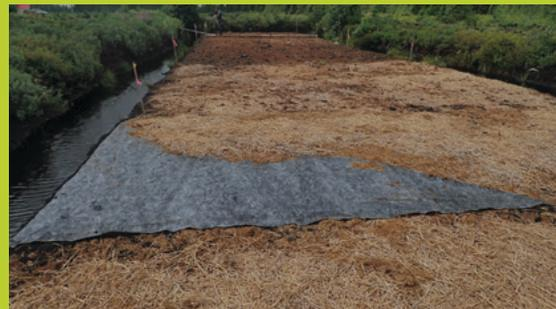
**Figure 28.** Plant material displaced by geotextile blown away by the wind.
