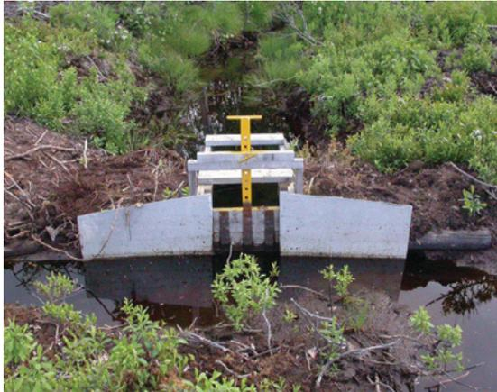
**Figure 15.** Fixed dam with manually adjustable level.
